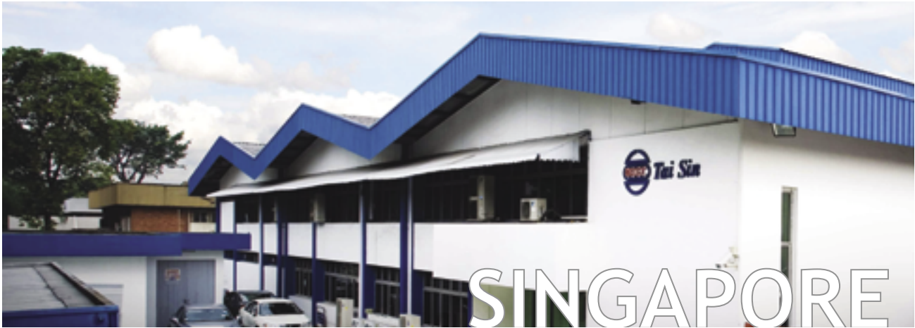
TAI SIN ELECTRIC LIMITED
