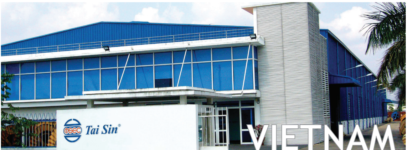
TAI SIN ELECTRIC CABLES (VIETNAM) CO LTD
